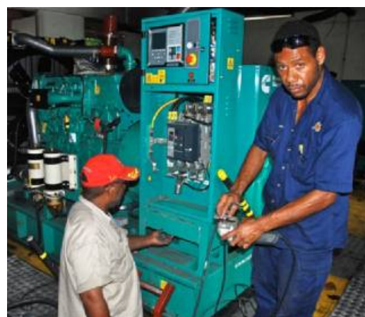
Biofuel Generator Installation Solomons
